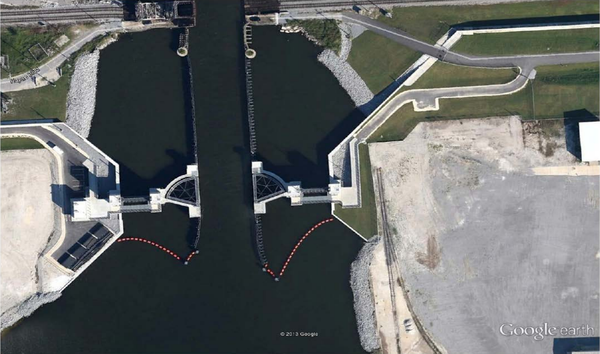
Figure 11. Lake Borgne Surge Barrier in New Orleans, Louisiana
