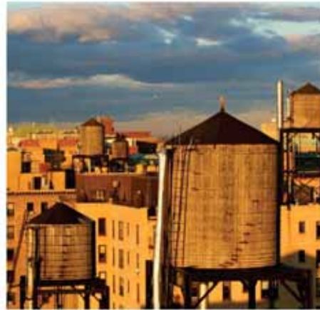
BR 8: Rooftop water towers have long been a fixture of the New York City skyline and, unlike pump driven systems, can help ensure access to potable water during a crisis.
